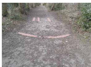
**32** The brickwork on the path indicates the location of the wheel pit at the top of the rope-worked incline. This was a self-acting incline with the weight of loaded bricks running down the incline hauling up returning empties. It was converted to locomotive operation in 1882.
